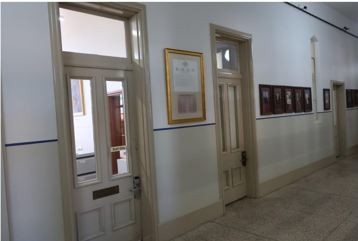
Figure 3.7 typical central corridor scene in the central building, ground floor, showing original door frames, door leaves altered with glass panels, and a c1950s triangular arched steel-framed window.
