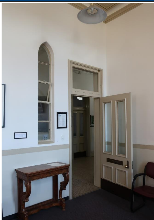
Figure 3.4 view from the ground-floor room Wilkinson Room towards the central corridor showing typical fenestration.
