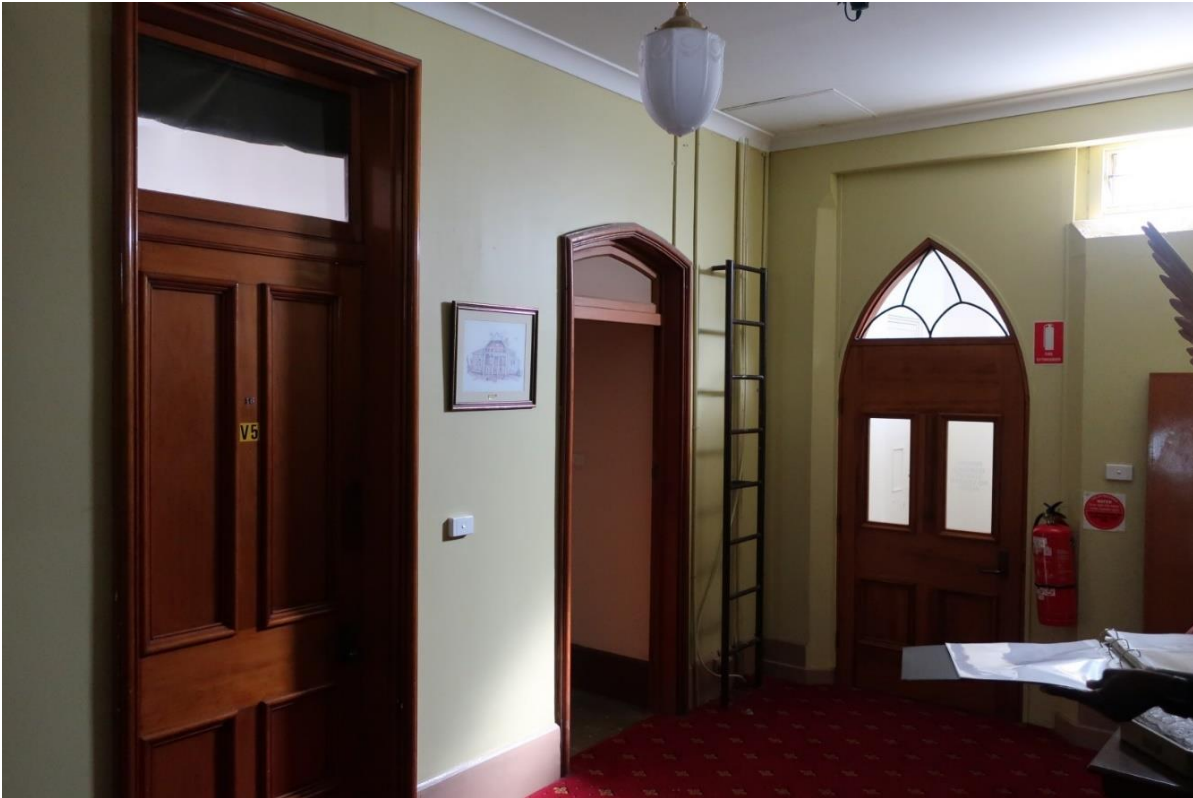
Figure 3.10 First floor inside the norther-western wing of the McAuliffe O'Reilly building showing two evidently original 1870s doors on the left and a modern one on the right. The choice of flat arch and pointed top-lights in the original windows likely indicated different room functions.
