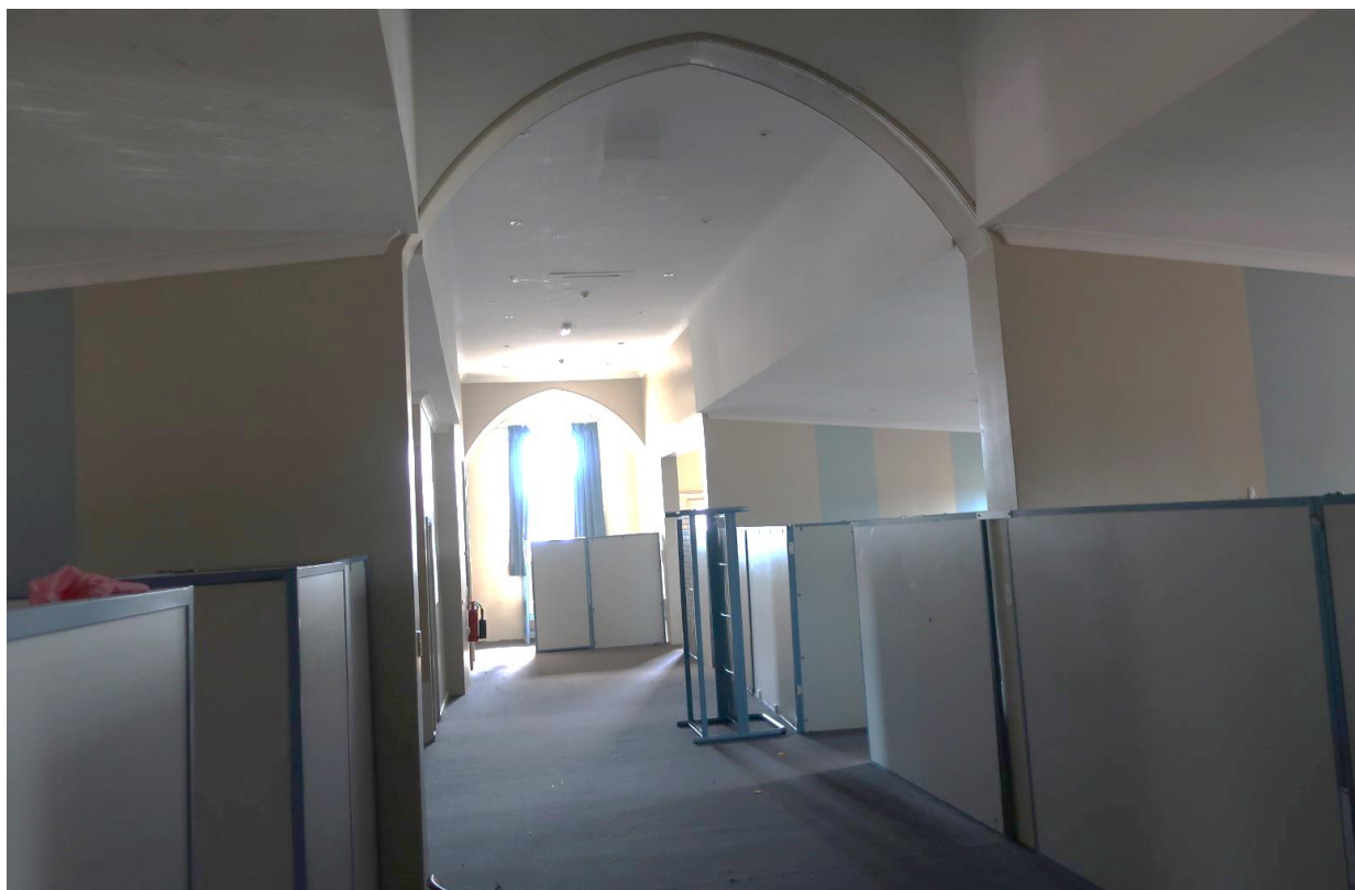
Figure 3.12 A boarding room on the second floor of the McAuliffe O'Reilly building. The staff mould around the arches seen here, and the window frames are the only decorated original finishes.
