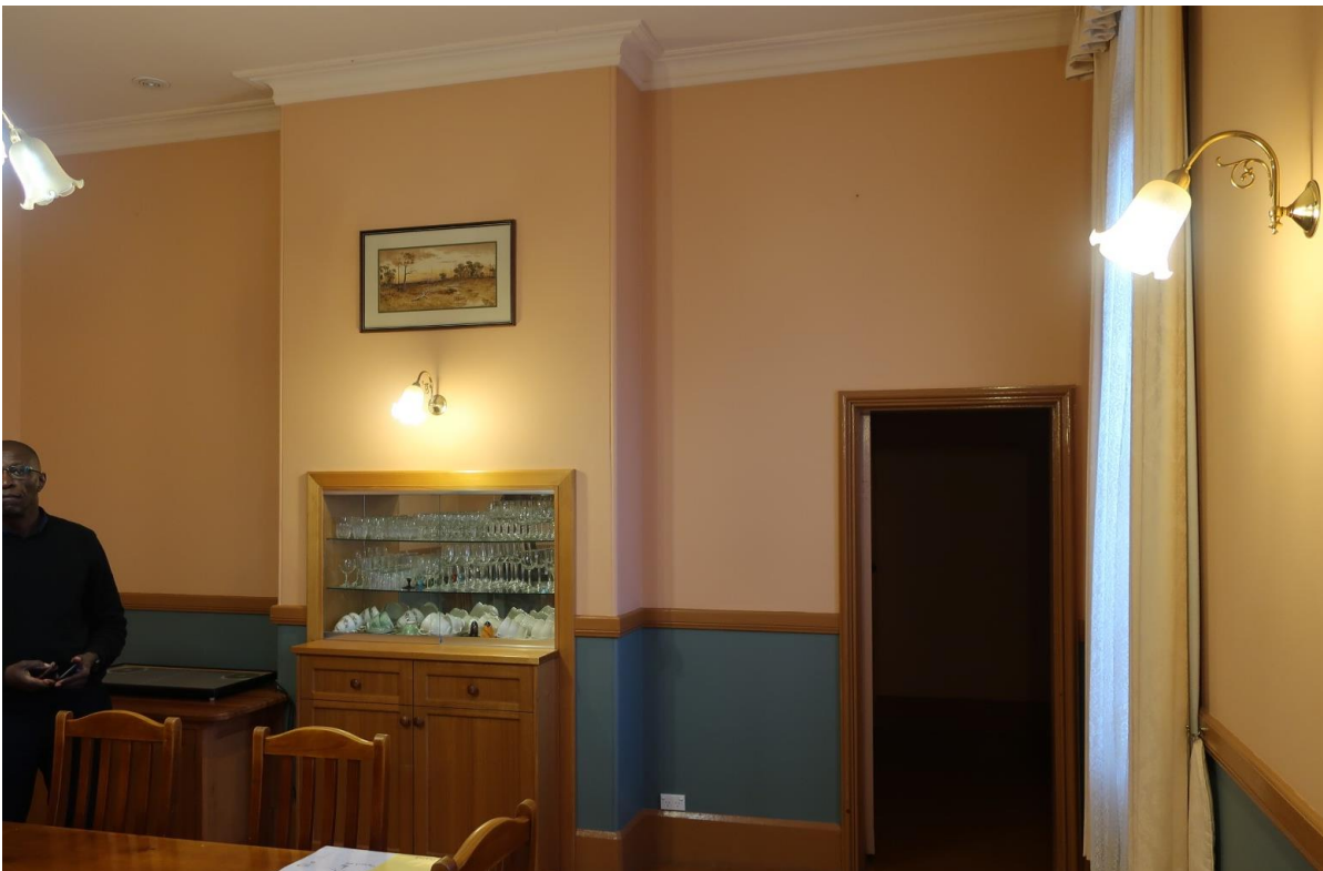
Figure 3.11 First-floor Vincentian dining room showing original door jamb, infilled fireplace with staff moulds, and Victorian style cornice.
